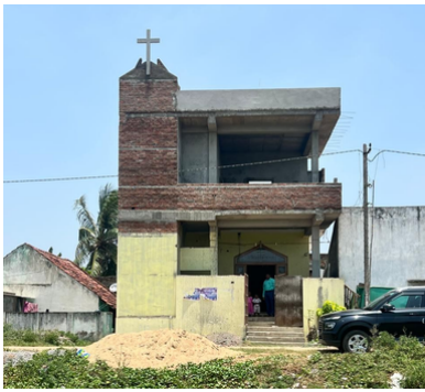
Upada Building progress
